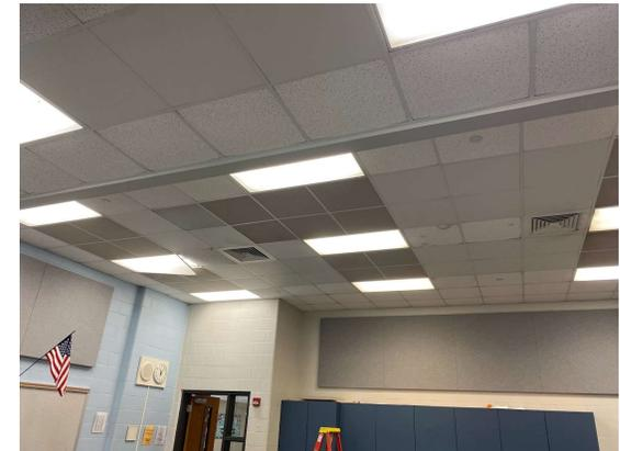
Examples of Wet Ceiling Tiles below AHU7/AHU8
